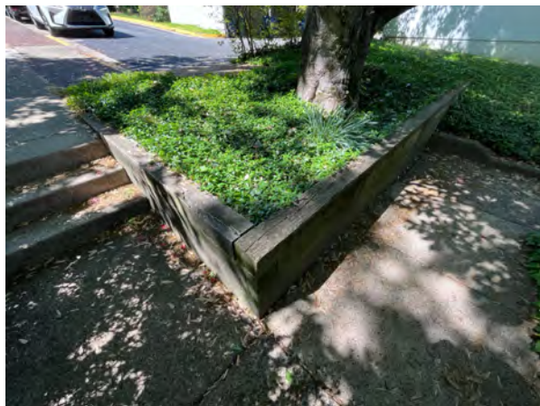
Association owned retaining walls are constructed of wood, brick and stone. Reserves budgets for brick and stone walls (long lasting components) to be repaired as needed. Top members of wood walls typically deteriorate first and they can be replaced to extend useful life; however, total replacement will eventually be needed. When replaced with a modular block system, they last longer and need less maintenance.
