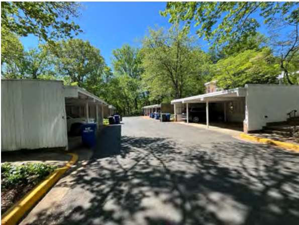
The association is responsible for 12 carport structures. Previous study included roof replacement based on varying age of roofs, an allowance for repair and replacement of roof drains and downspouts, and wood siding replacement. Association is planning a repair/restoration project in FY26. See "Comments" section for study assumption for this work.
