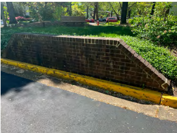
Association owned retaining walls are constructed of wood, brick and stone. Reserves budgets for brick and stone walls (long lasting components) to be repaired as needed. Top members of wood walls typically deteriorate first and they can be replaced to extend useful life; however, total replacement will eventually be needed. When replaced with a modular block system, they last longer and need less maintenance.
