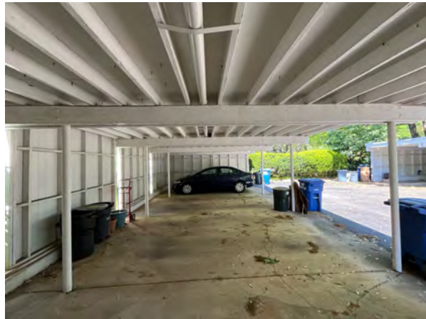
The association is responsible for 12 carport structures. Previous study included roof replacement based on varying age of roofs, an allowance for repair and replacement of roof drains and downspouts, and wood siding replacement. Association is planning a repair/restoration project in FY26. See "Comments" section for study assumption for this work.
