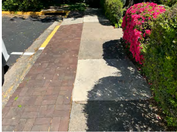
Community curbs, gutters and sidewalks are Association responsibility. Reserve provides for these components to be repaired as needed.
